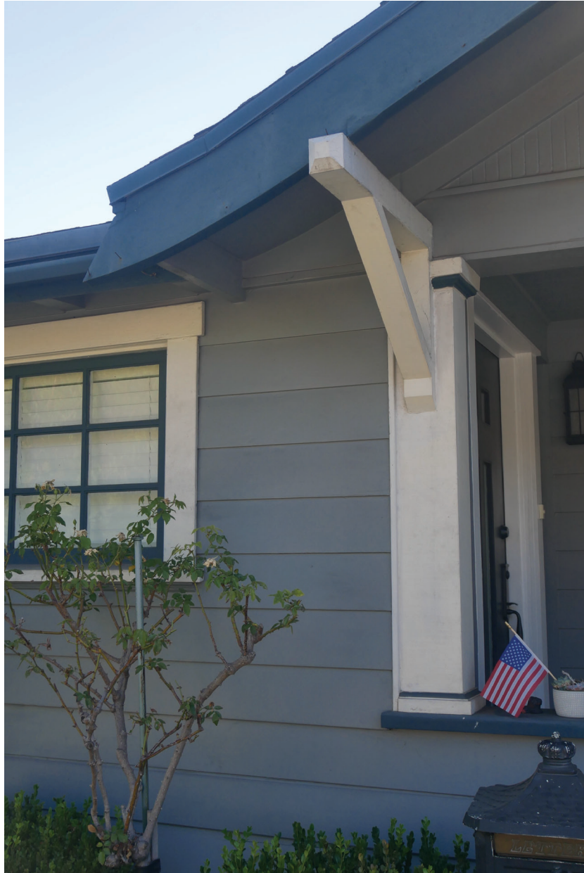
Photograph #7: Porch gable roof knee brace
