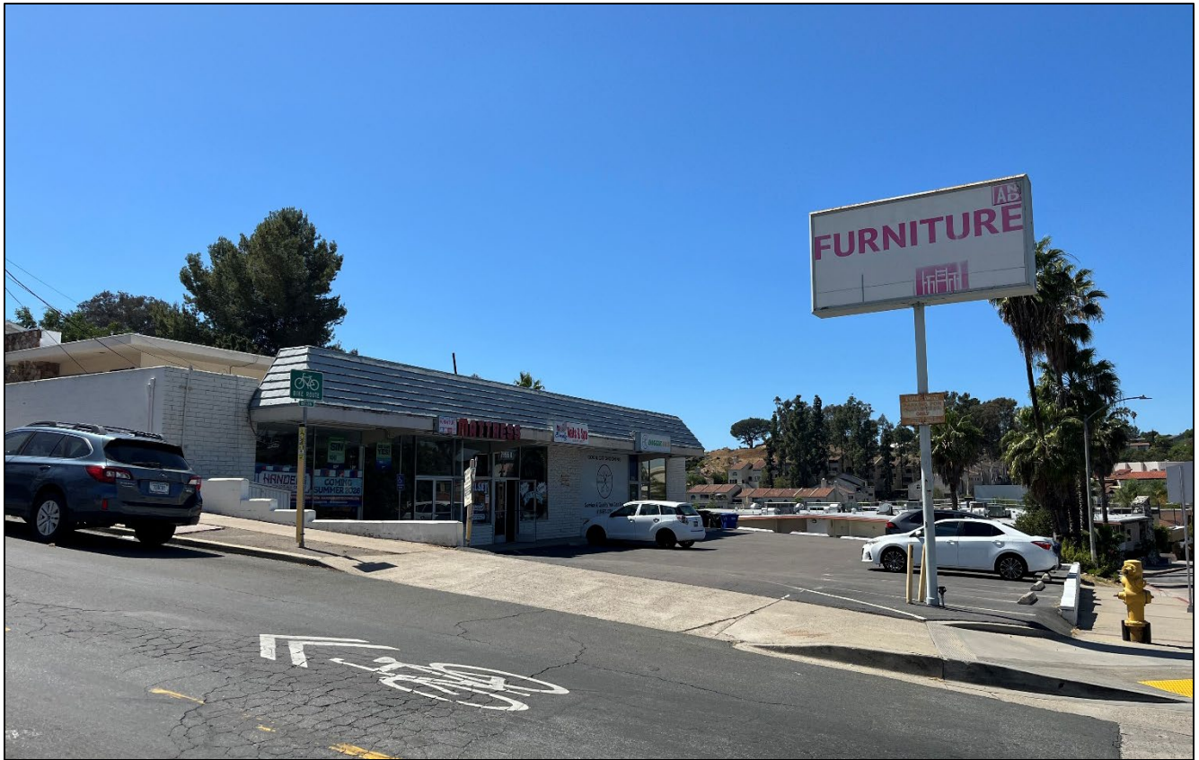
Existing Northeast Façade facing west
