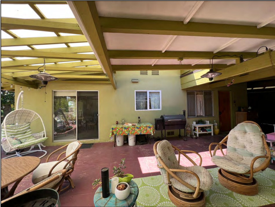
Photo 10e: Detail view west of covered patio. Vinyl window is visible Source: Urbana Preservation & Planning.
