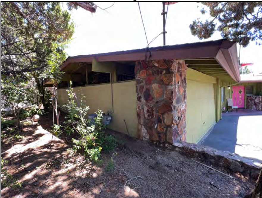
Photo 8a: The east elevation faces neighboring property 9361 Lemon Avenue. The elevation has a concrete block wall with a custom cut stone veneer on the north corner and adjoining stone wall, a wide eave overhang with rafter exposed beams, an open space below the main roofline and the concrete block wall, covered with a metal mesh, and minimal decorative details. Source: Urbana Preservation & Planning, LLC.
