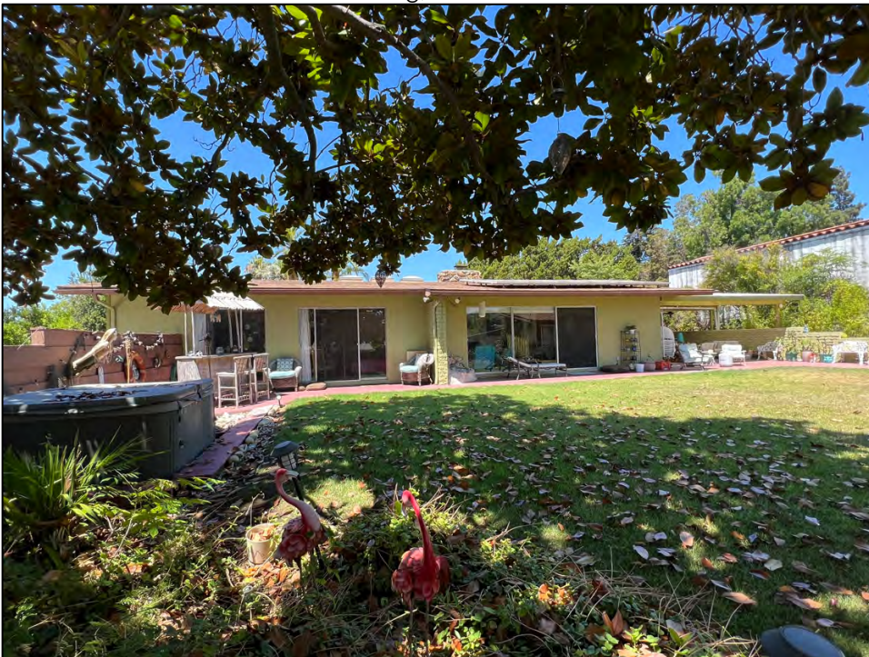
Photo 9b: The elevation features a stucco façade, large aluminum sliding glass windows, a partially covered patio on the southeast corner, and a partition wall separating the bedrooms from the common space areas.
