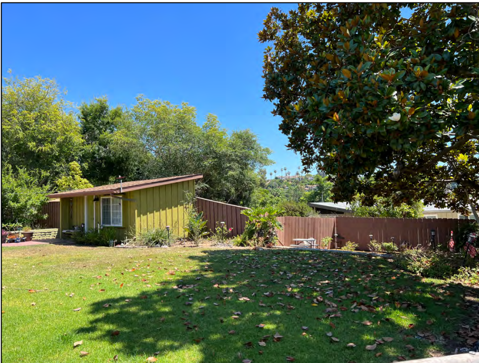
Photo 11: Directly south of the main residence is a wood-framed "tool and storage" ADU that was constructed in a similar style with board-and-batten siding, and a slightly pitched shed roof with moderate eave overhang. Source: Urbana Preservation & Planning.
