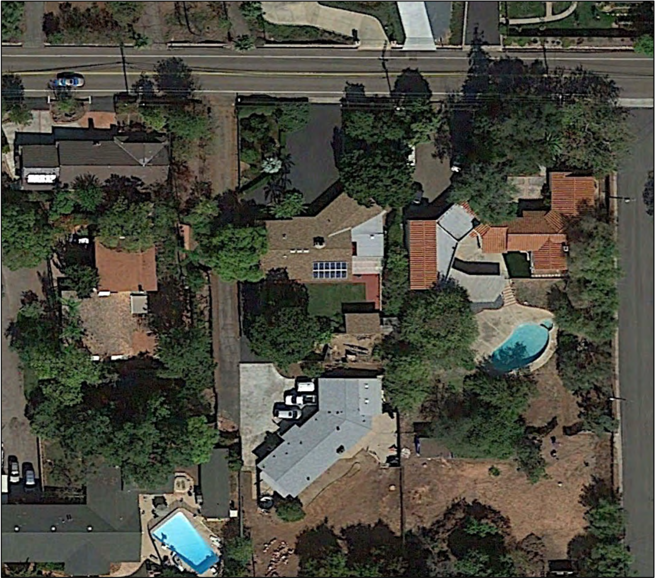
Figure 31h: Aerial view of the subject property, 2012. Between 2010 and 2012, original roofing over the covered patio on the southeast corner was removed and corrugated roofing was added and extended north on the garage area. Source: Google Earth
