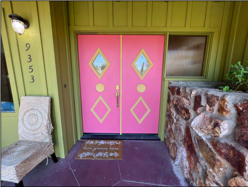
Photo 3: The elevation is crescent shaped, asymmetrical, and partially obscured from the public right-of-way by vegetation along the road. The main entryway is mostly centered and recessed below the main roofline and features two Mid-century style doors painted in pink with diamond lite windows. Custom cut stone planter is visible to the left of the main entryway. Source: Urbana Preservation & Planning, LLC.
