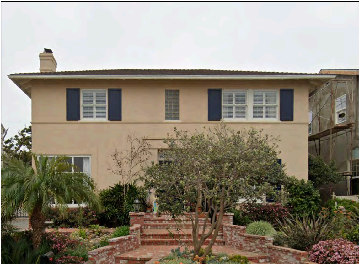
Figure 17b: Street view of the 3319 Udall Street property. Source: 2020 Google Street View
