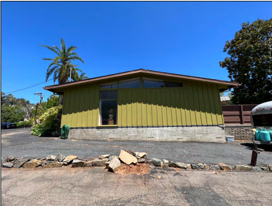
Photo 7b: The elevation has an asymmetrical façade and features board-and-batten siding, clerestory windows installed at the gable end, a wide eave overhang, a single louvered window above a large rectangular frameless frosted window, concrete block along the lower span of the dwelling, and minimal decorative details. Source: Urbana Preservation & Planning, LLC.
