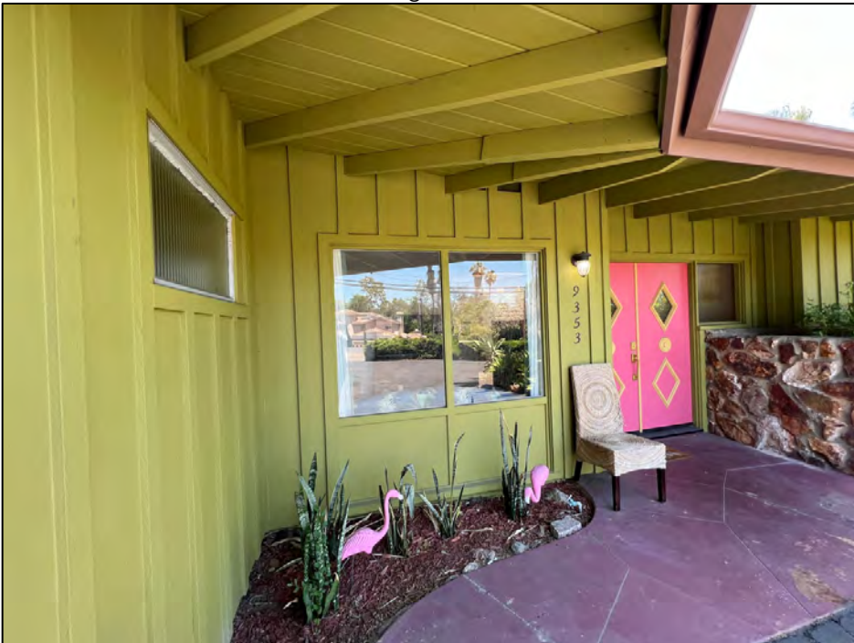
Photo 4: To the east (left) of the front door are two large double fixed frameless windows, with wood panels on the lower half. The wood panels replaced original louvered windows that are visible in the original drawings. Source: Urbana Preservation & Planning, LLC.
