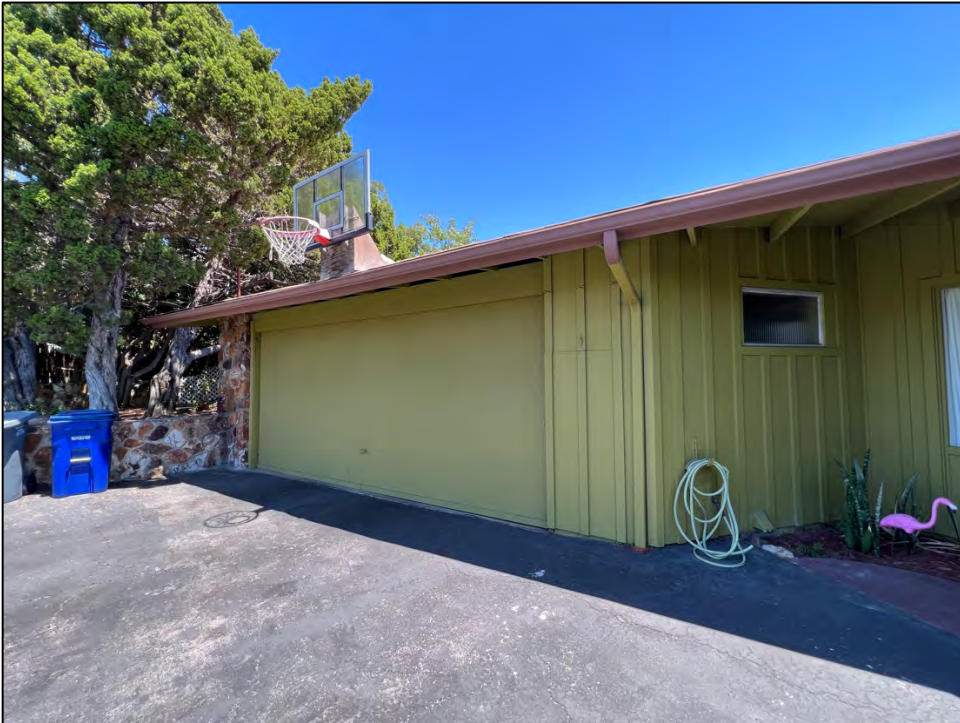
Photo 5: The double-car garage is located to the far east end of the elevation and features board-and-batten façade, a wood overhead door, and a single aluminum frosted glass window. The custom cut stone wall is visible in the photograph. Source: Urbana Preservation & Planning, LLC.
