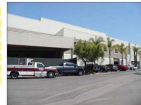
EDCO facility located in the industrial center.
