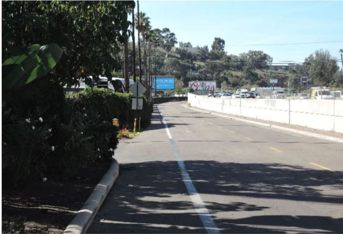
Figure 37 - Lack of Street Improvements on South Side of Road
