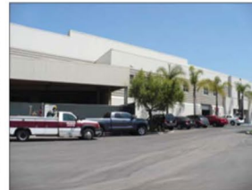
EDCO facility located in the industrial center.
