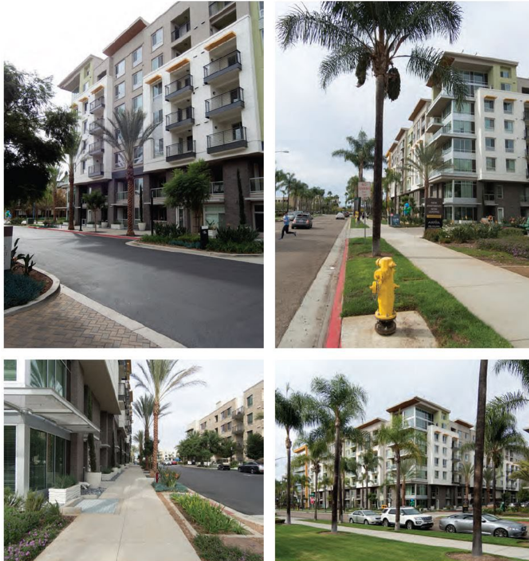
Figure 17 - Liner Unit Examples - Photos
