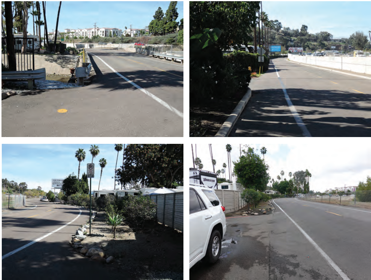
Figure 27 - Photos Showing Lack of Standard Public Improvements on the Alvarado Road Frontage
