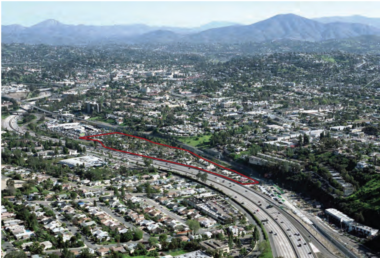
Figure 1 - Aerial View of the Specific Plan Area
