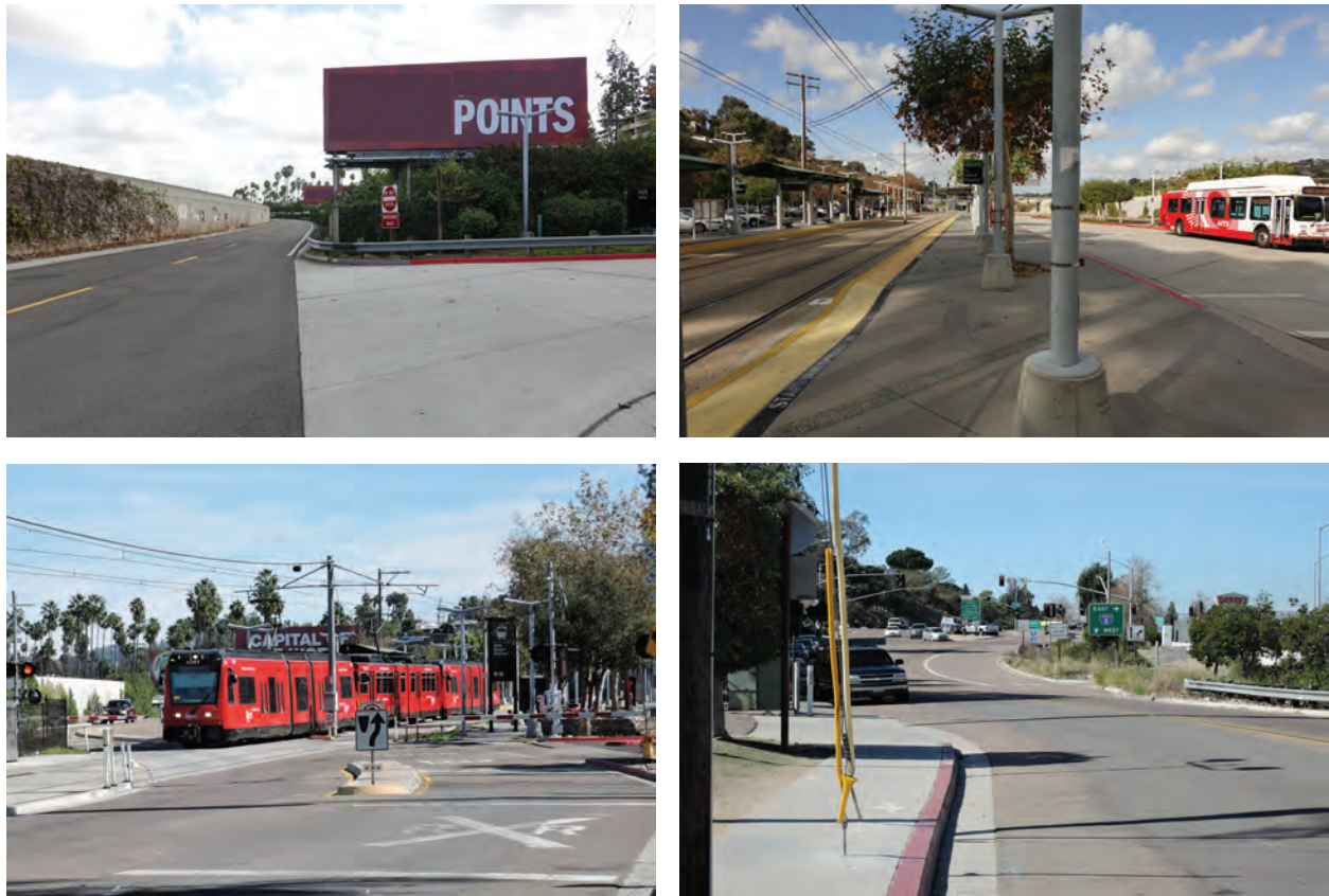
Figure 9 - 70th Street MTS Station, Existing Conditions
