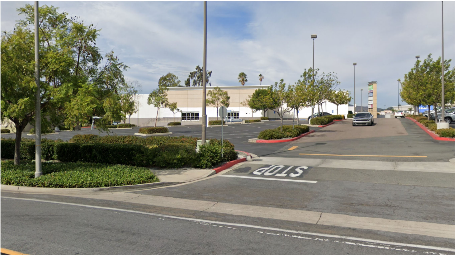
View of project site from Grossmont Boulevard
