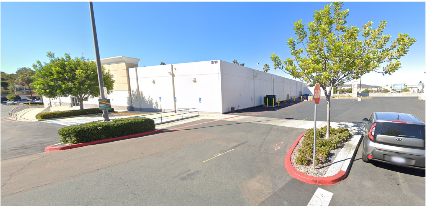
View of project site from parking lot looking northwest.
