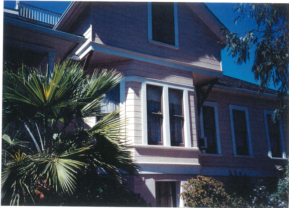
Wall dormer over angled bay on east side.
