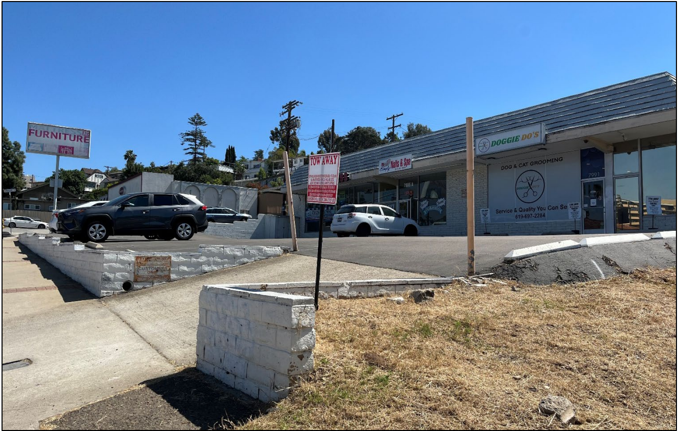
Existing Northeast Façade facing south
