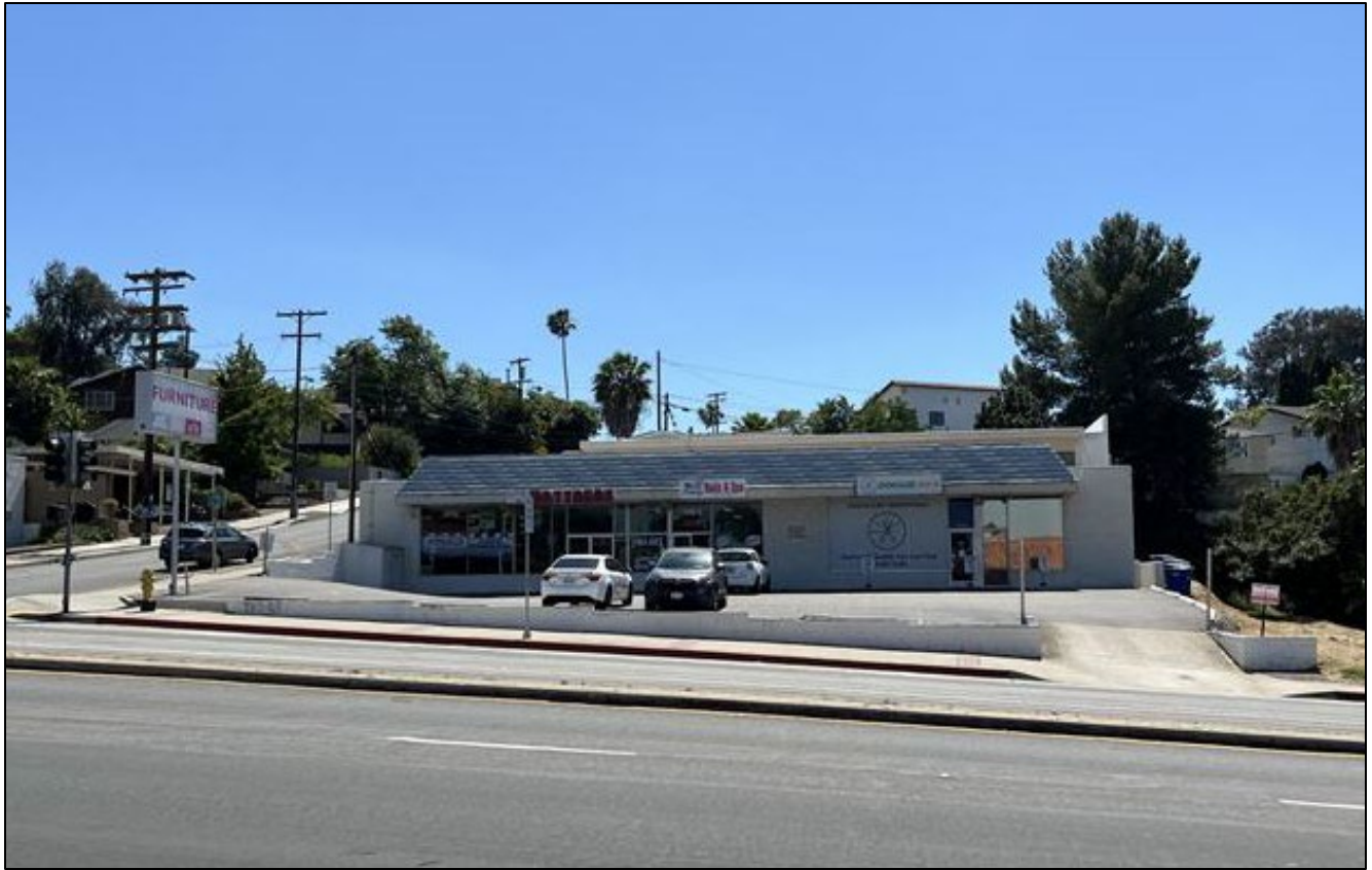
Existing Northeast Façade facing southwest
