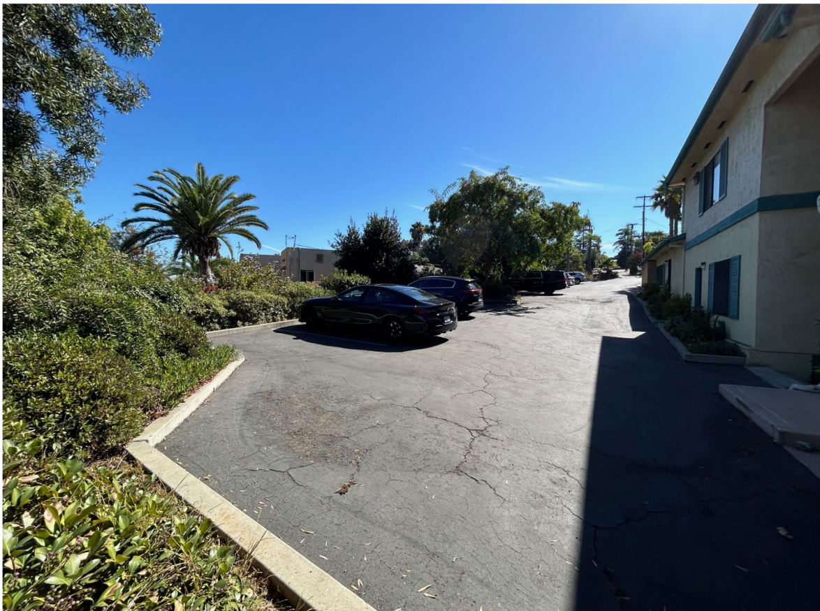
Parking area at the north end of the site, looking southeast.
